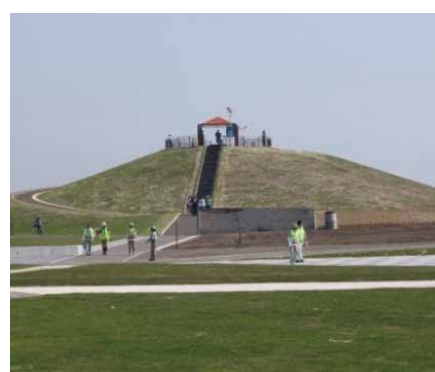
(6) Construction of Artificial Hills
